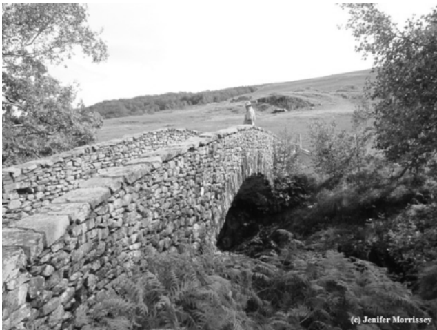
The rebuilt packhorse bridge in Wet Sleddale [another photo in the Colour section]
